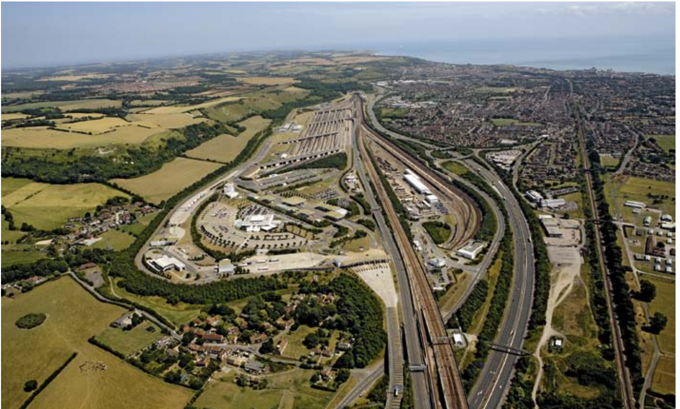
UNDERSEA RAILWAY: The Folkestone Terminal on the British side of the Channel Tunnel, with the tunnel mouth in the centre of the picture and the English Channel in the background to the right.
